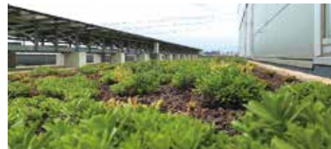
107.5 m 2 of rooftop greenery to reduce AC power consumption (R&D Center)
