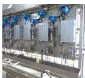
Boiler sampling system installed at a biomass power plant
