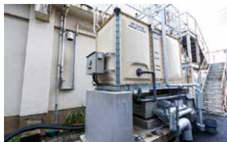
Wastewater from reverse osmosis water purification reused for toilet flushing (Saitama Factory)
