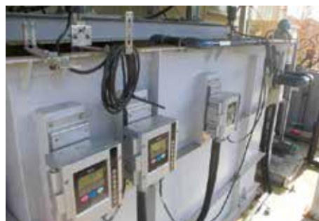
pH neutralization facility (Saitama Factory)
